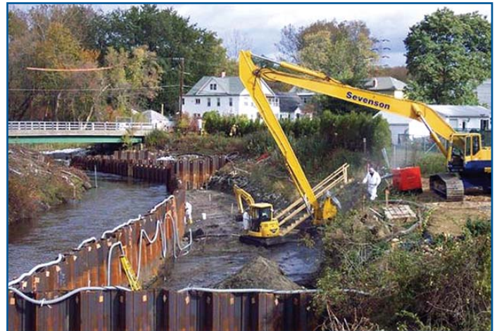
Removal – Excavation in the “Dry”
